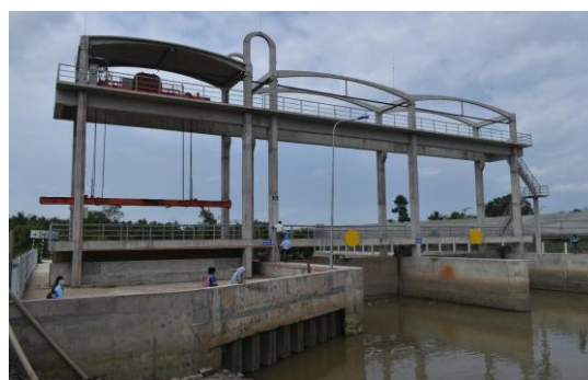
Figure 4. Bai Dac sluice gate constructed in 2020
