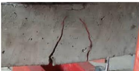
Figure 5. Pictorial evidence of flexural failure of test beam
