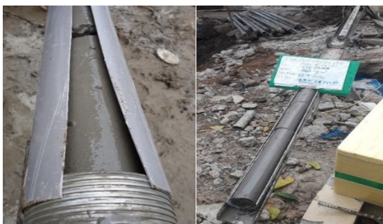
Figure 5. Drilling SCM cores and determining quality
