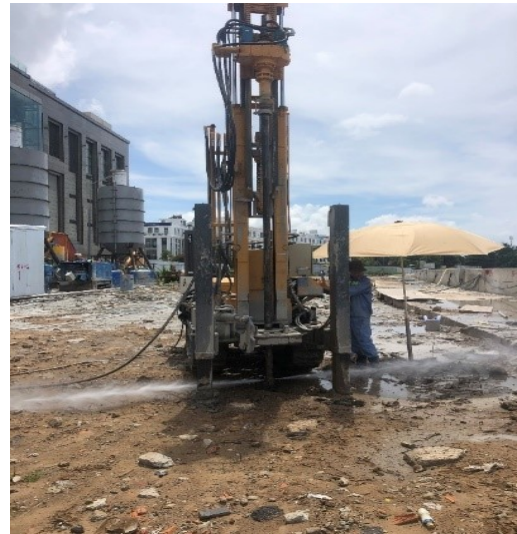
Figure 6. SCM by Jet-grouting method
