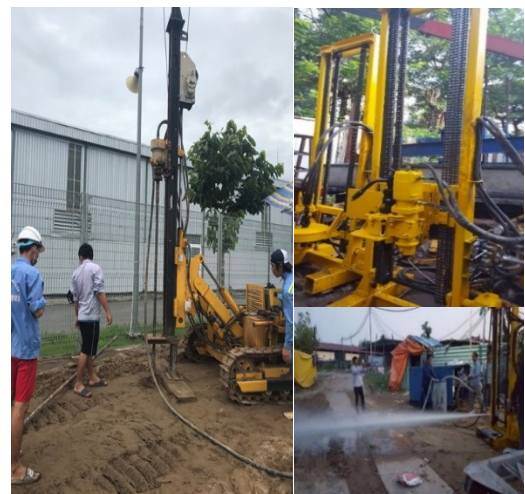
Figure 4. Drilling system used in the study
