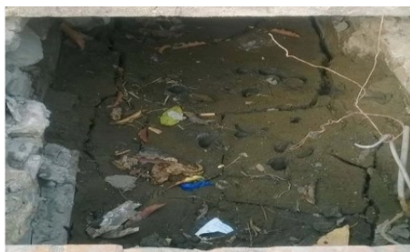
Figure 5. A manhole on Phan Dinh Phung street
