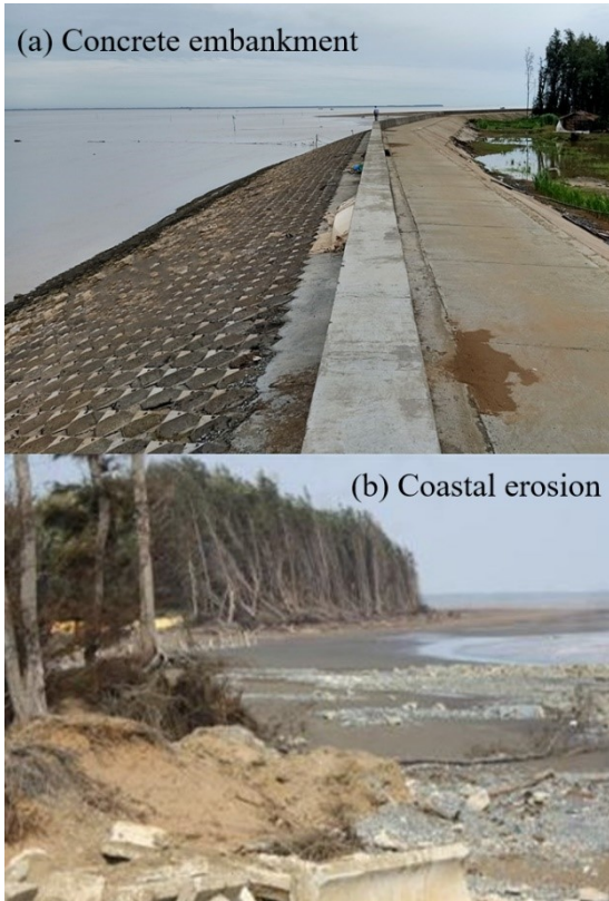
Figure 2. The embankment and coastal erosion as depicted as yellow rectangle and red circle in Figure 1
