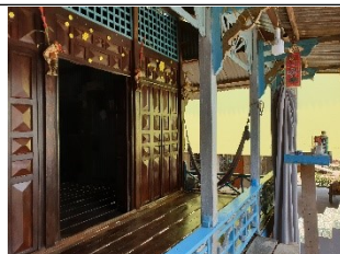
View of verandah
